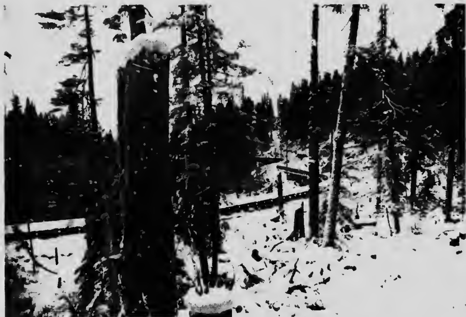
Granby Consolidated Mining, Smelting and Power Company Limited. 72 Inch Wood Stave Pipe Line under Winter conditions.
